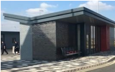
Figure 2-2: EMG1 Bus Interchange
